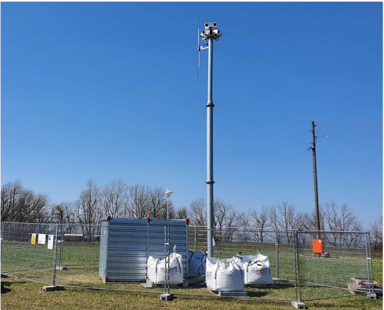
Illustration 1: Installed IDF system with a mast height of 10 m.
